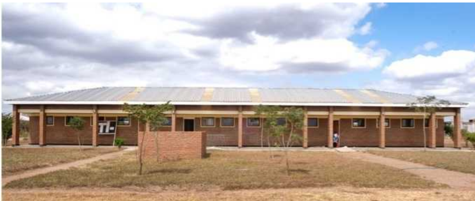
Classroom building at Kuwala Christian Girls School in Malawi
